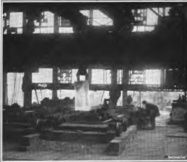
Fig. 4. Lowering a Steel Ingot into a Blooming Mill Soaking Pit for Reheating Prior to Rolling
